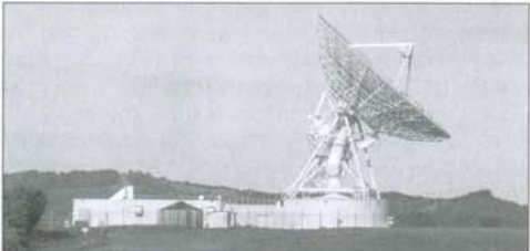
ZM2TV on 5.7GHz EME with 30.5m dish
